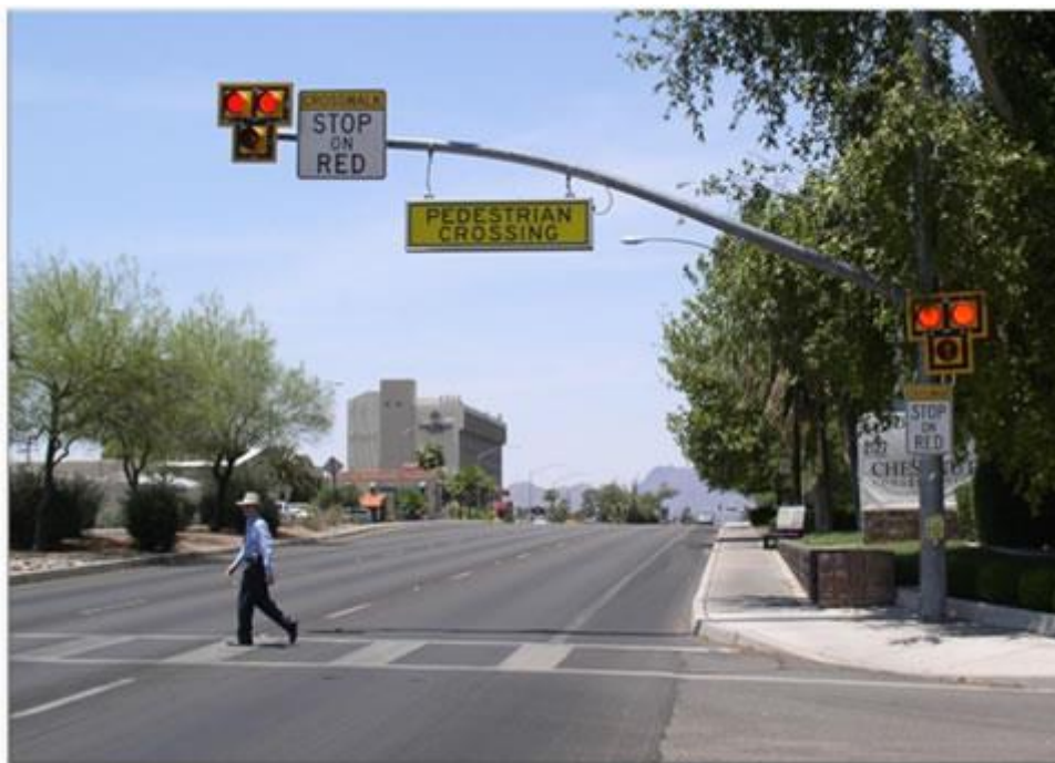
Example of a HAWK treatment in Tucson, AZ
